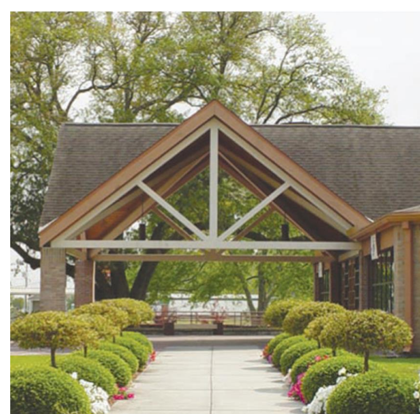
Figure 1: Examples of Planar Trusses in Roof Systems [1]
